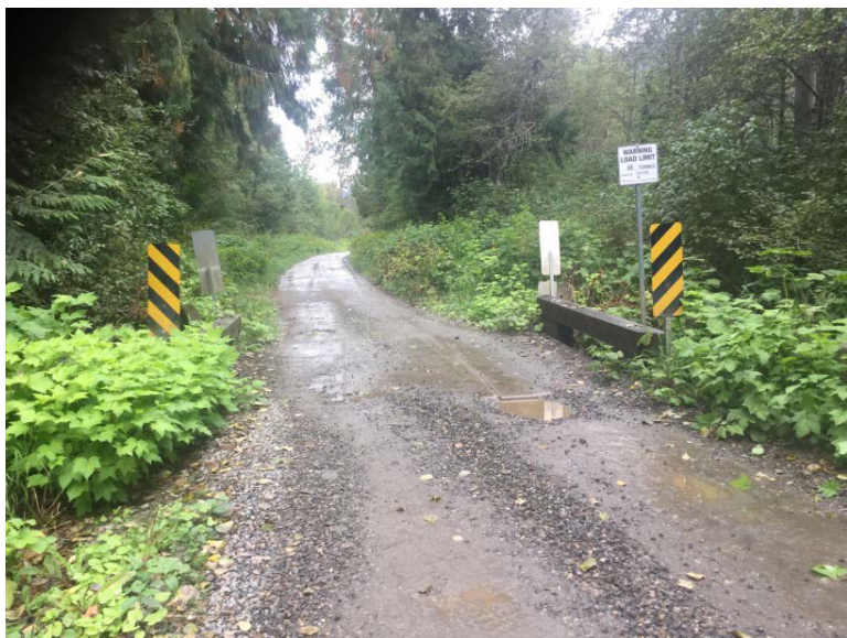
Approach from Right Bank when facing downstream
