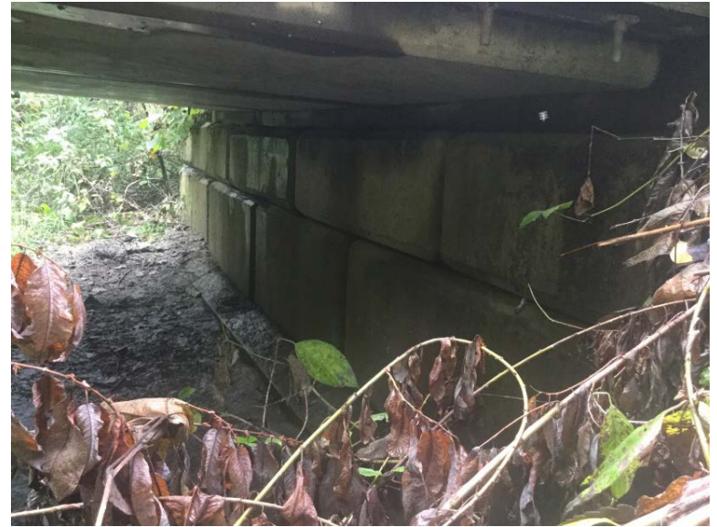
Right Bank Abutment when facing downstream
