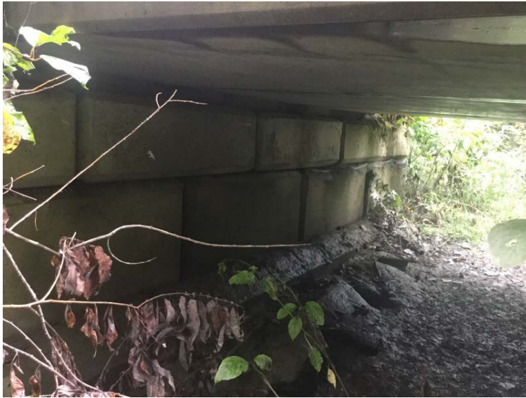
Left Bank Abutment when facing downstream
